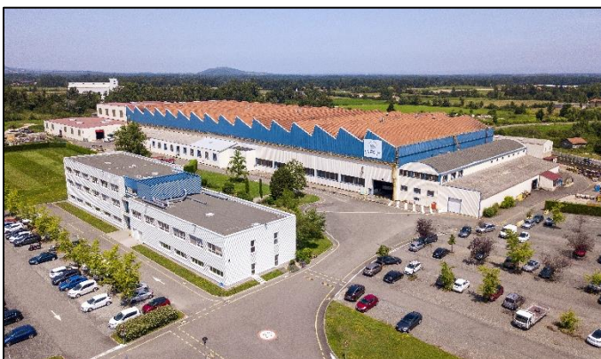
Figure 11 – Clecim SAS (Montbrison city, France)
