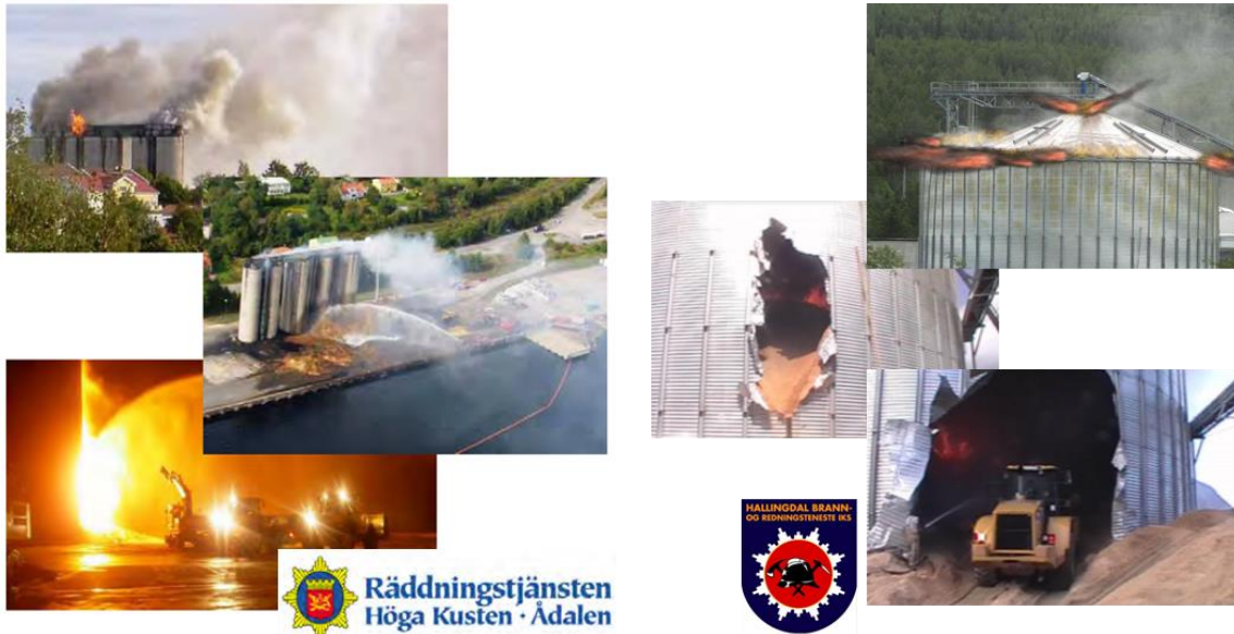
Figure 2: Consequences of Oxidation. Left, Silobrand Härnösand [8-13 Sept 2004]. Right, Hallingdal Trepellets [10 July 2010]. These are just a couple of the reported incidents that occurred in wood pellet silos where self-heating lead to ignition.
